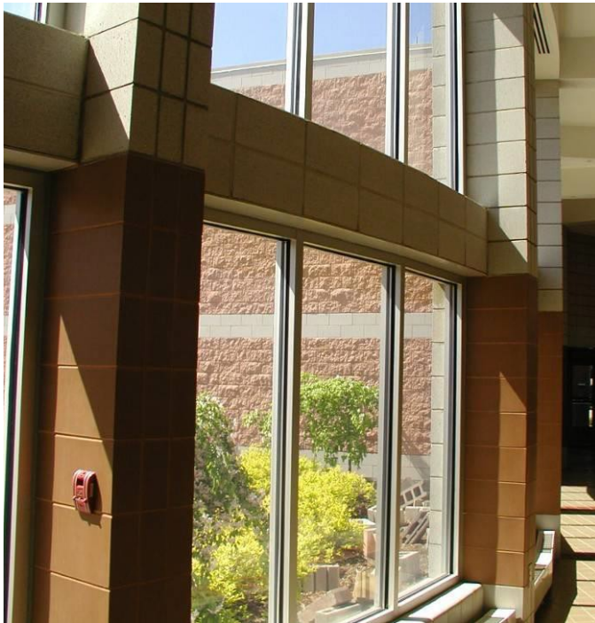
Concrete block between upper and lower windows allowing water infiltration – flashing is suspect.
