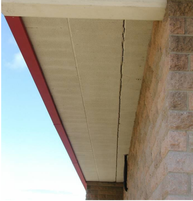
Concrete plank roof shifting at Besser Technology Center – connecting cables are suspect.
