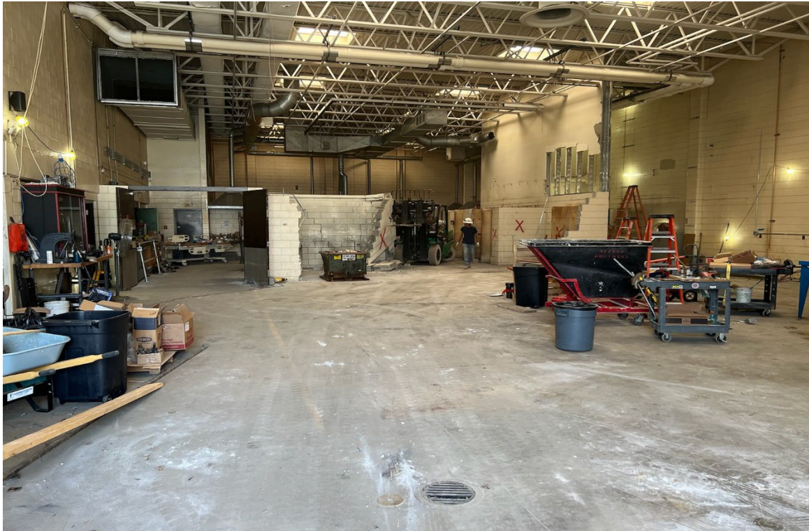
ACC Welding Lab without manufacturing equipment and partition wall (June 14, 2023).
